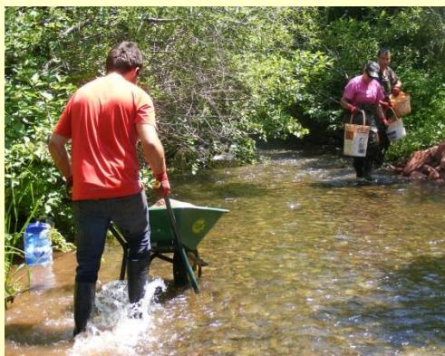
CBWA identified an erosion issue on a waterway at Marchbanks. The bank was degraded, disrupting the normal flow pattern. With the assistance of students from the STARS program, CBWA staff re-established the bank with rocks and filter-fabric - therefore re-directing the stream flow and deepening the channel. We want to extend a sincere thank you to the STARS group - the students braved the bugs and the hot summer temperatures to complete the job.
